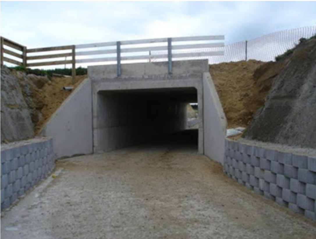
Open-arch culverts work very well as wildlife feel safer entering a large opening
