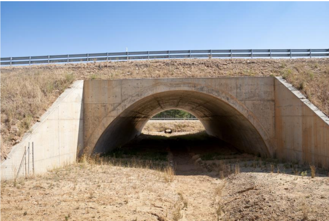
Open-arch culverts work very well as wildlife feel safer entering a large opening
